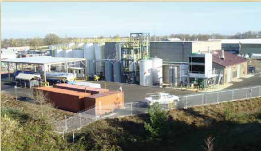
Figure 1.5a Sequential Pacific Biodiesel in Salem, OR is an example of a diversified biodiesel plant which utilizes soybean oil, canola oil, and waste cooking oil to produce over 5 million gallons of ASTM specification biodiesel each year. This fuel is blended with petroleum and sold in Oregon, Washington, Idaho, and California.
