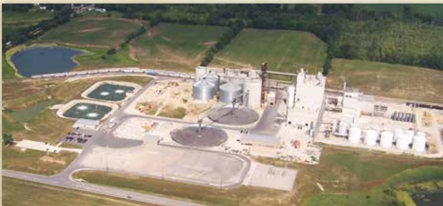
Figure 1.5b Louis Dreyfus Biodiesel plant, located in Claypool, Indiana, is the largest integrated soybean/biodiesel processing plant in North America. The annual capacity for biodiesel production is 88 million gallons/year. This is a BQ9000 certified plant, which ensures high quality product/processing at each step in the manufacturing process.
